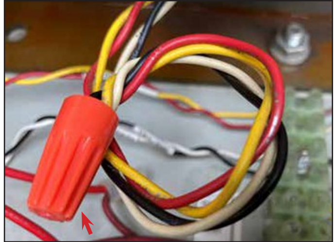
Figure 12 Cut BMID Wires Screwed into One Wire Nut
