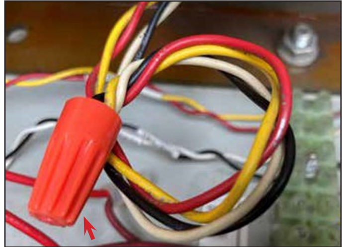
Figure 20 Cut BMID Wires Screwed into One Wire Nut
